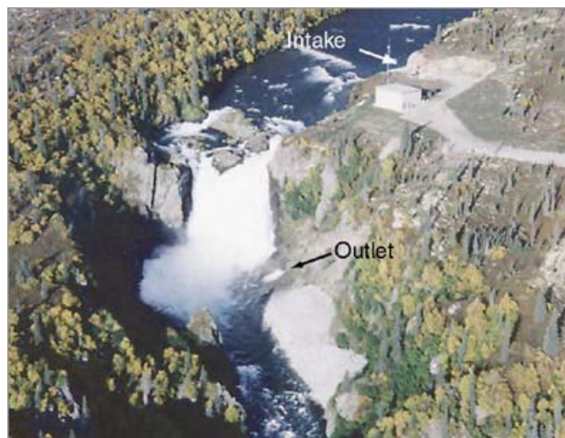
Figure No1. The Tazimina project in Alaska is an example of a diversion hydropower plant. No dam was required
