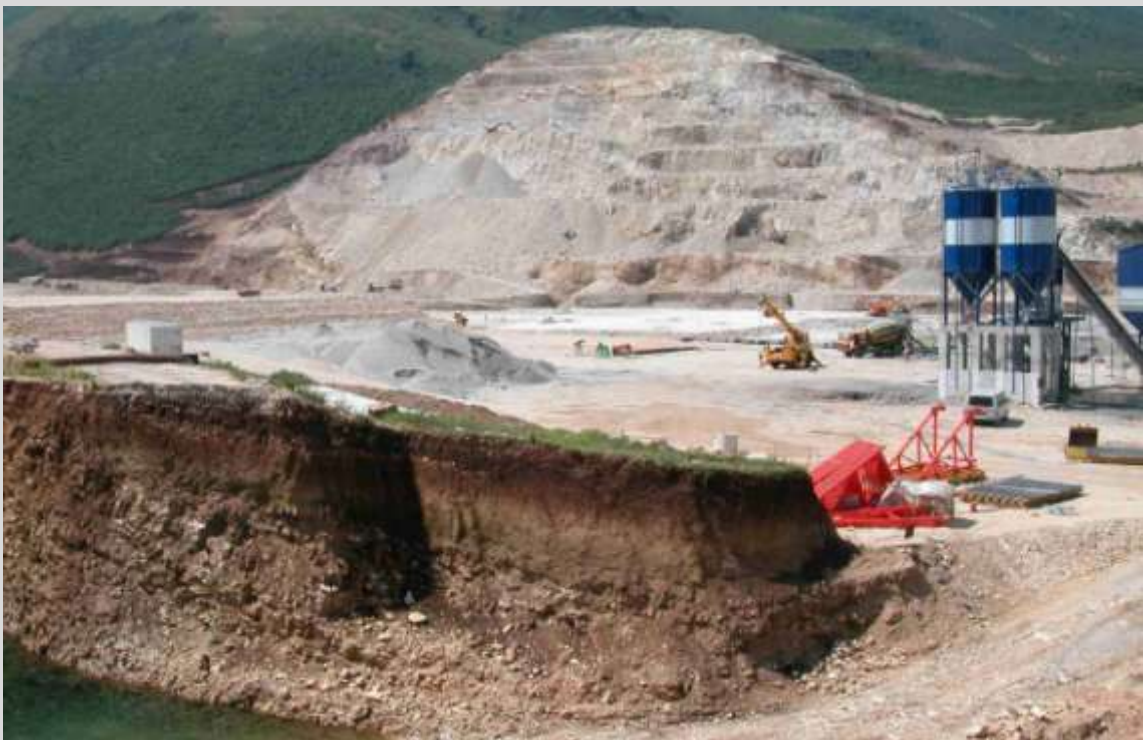
Construction works of Kalivac Dam in 2008 (Arno Mohl, WWF Austria).
