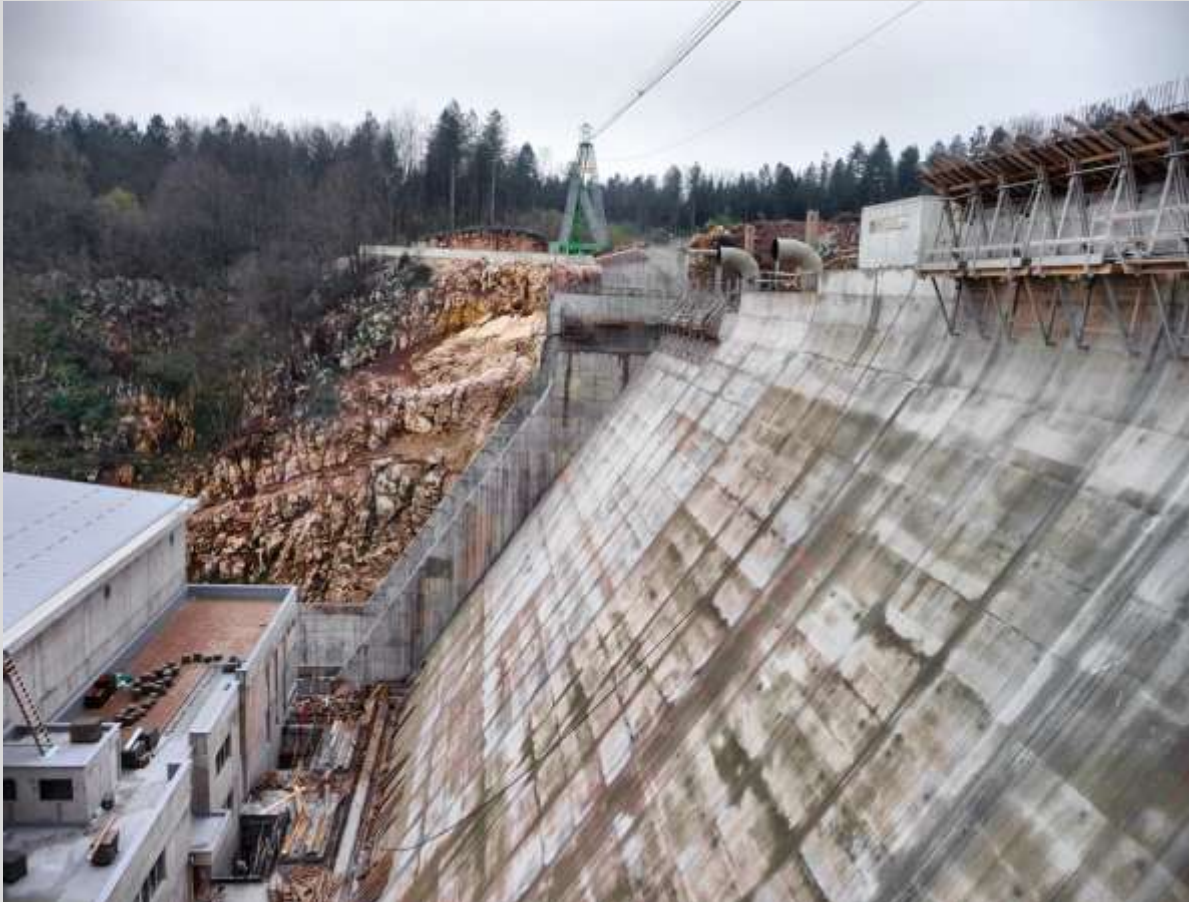
Construction works in 2008 (Google Panoramio, by user haze 2005).
