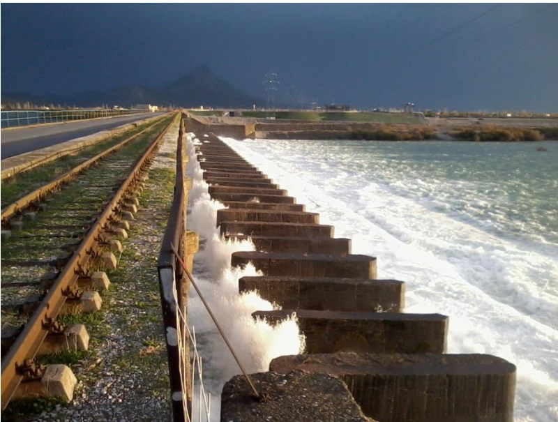
Movable Weir at Spathar, Drin
