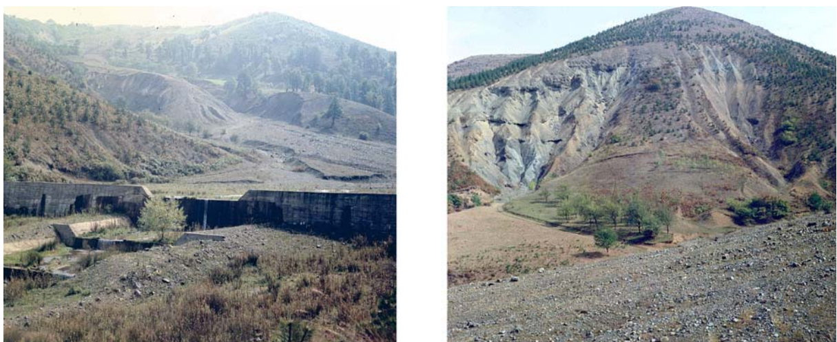
Figure 13. Check dam and combination of counter-sloped and normal protective forestation
